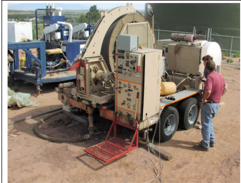
Fig. 12. Coiled tubing unit and mud system drilling on the ridge at the San Ysidro, NM site.
